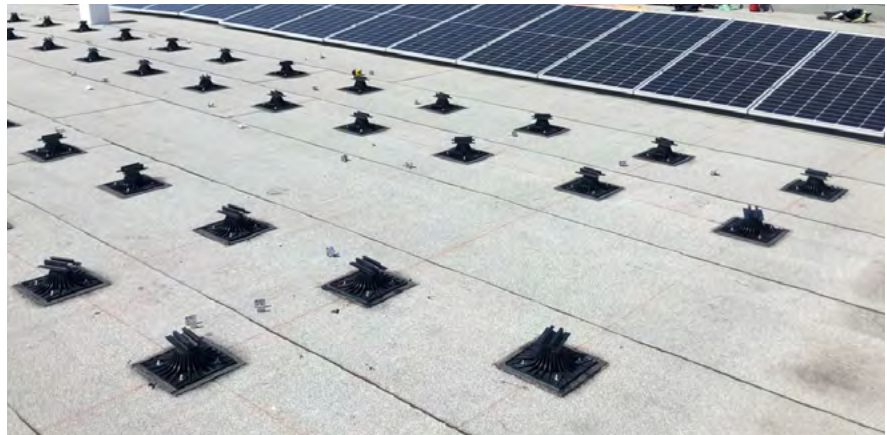
Weld the other side of the base panel over a minimum width of 3 cm.
