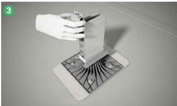
3 Insert the cage nut of the support clamp kit in the raiser through the opening provided.
