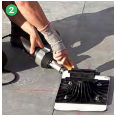
Weld the other side of the base panel over a minimum width of 3 cm.
